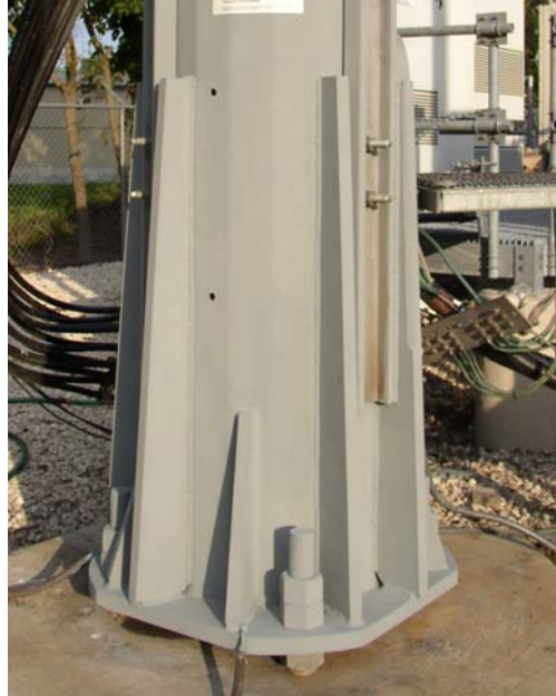
Map Tower, Clean and Grind. Prepare Surface for welding.
